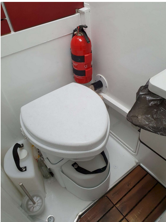
Dry separation toilet
